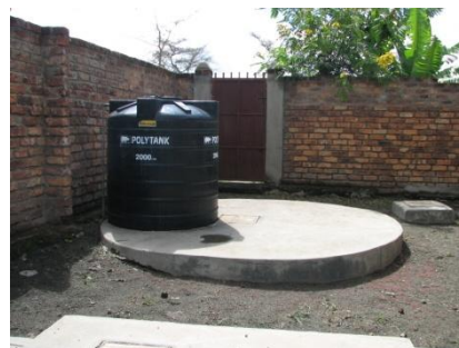
1 of 2 water tanks
