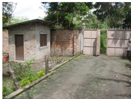
Entry gate & store
